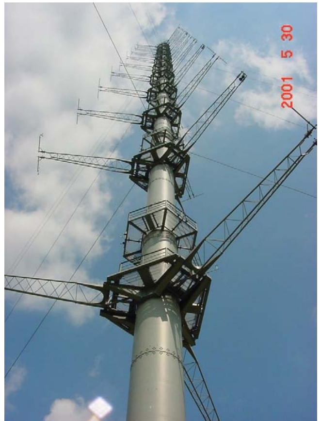
Figure 2: The 213 m meteorological tower with its booms at 20 m intervals. Three different boom direction can be exploited to avoid mast interference. Booms can be put in vertical position for instrument maintenance
